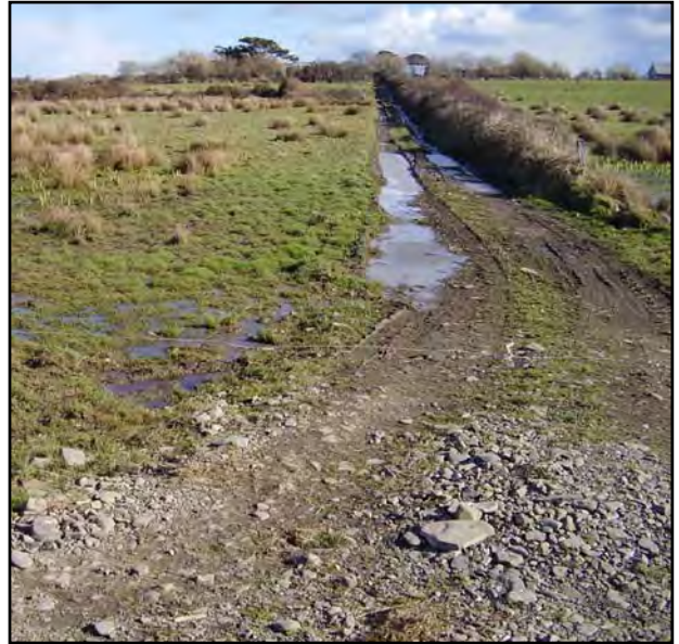
No. 34 – Water pooling along road at base of D8 near beach (D8-SW2) at GPS: E101341, N148335.
